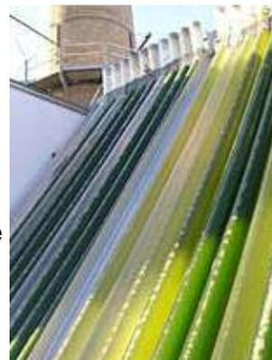
Smokestack emissions bubble through algae-filled tubes at MIT's Cogen plant.. (Photo: Ashley Ahearn from [www.algae4oil.com](http://www.algae4oil.com))
